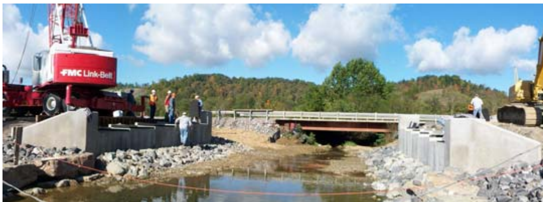
Abutment 1 (left) used SCC for its three caissons, while Abutment 2 (right) used a traditional caisson mix.
