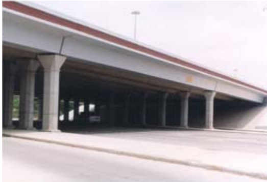
Louetta Road Overpass, Houston, TX Issue No. 1
