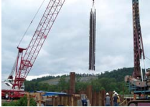
Reinforcement cage being lowered into place.
