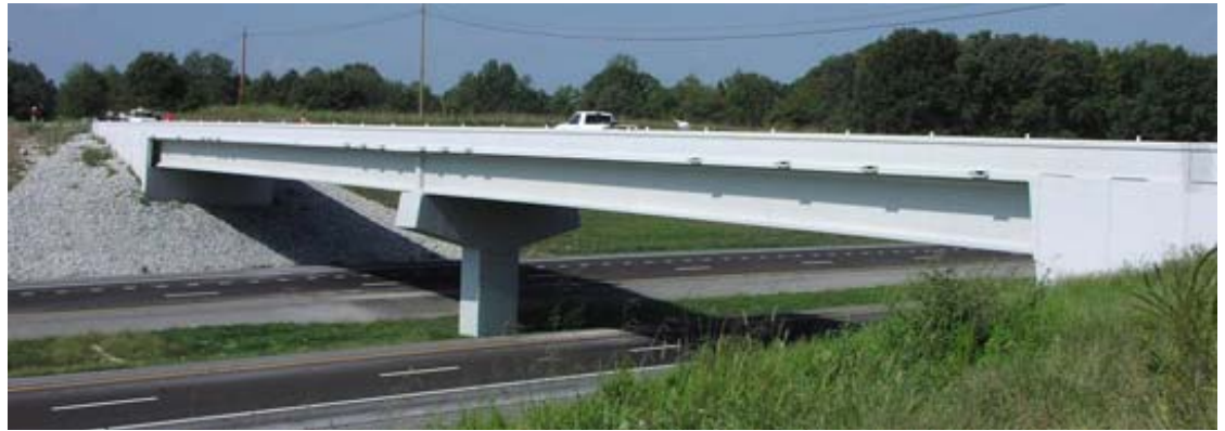
HPC was used in the superstructure of the Hickman Road Bridge, TN
